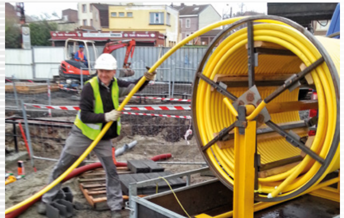
Installation of pipe LPG-FLEX
