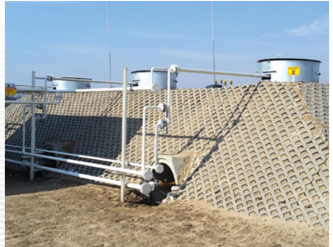
Project LPG Distribution Facility: 3 x 50 m 3 , Ø 2500 mm
