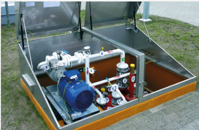
Project Module LPG at the Petrol Station
