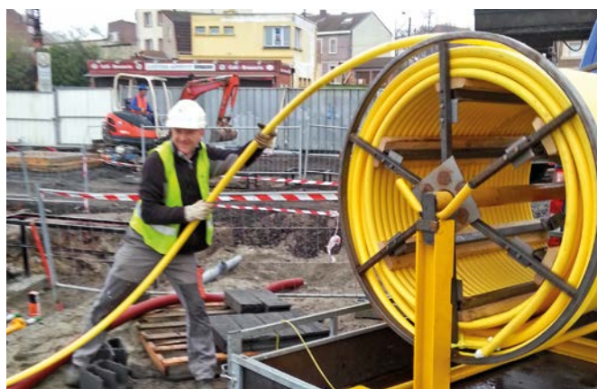
Installation de tuyaux LPG-FLEX
